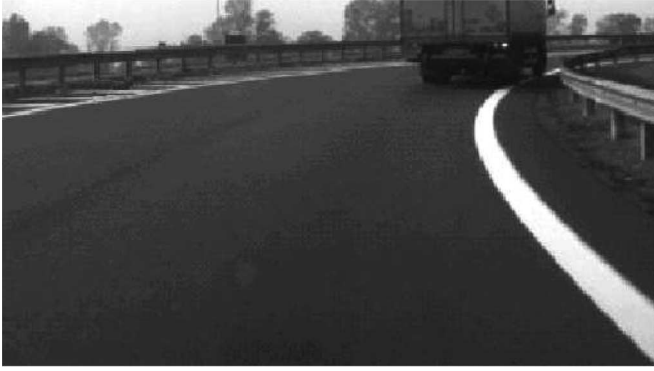
Fig. 22. Beltway. Guard rail is almost horizontal and is not identified.
